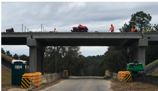
Crews placing deck pans on bridge over Rodgers Rd.
