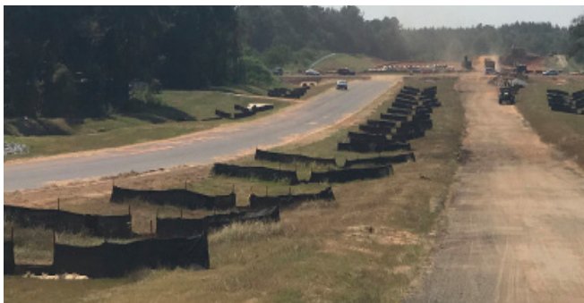
SR-158 extension west of Stone Rd.
