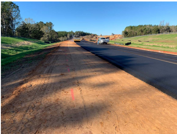
Crews grading shoulder at SR-158 extension or the Stone Rd. interchange.
