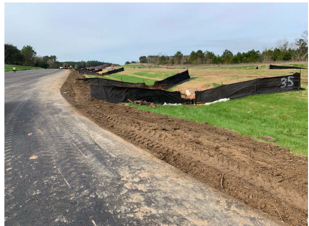
Topsoil placed for SR-158 extension shoulders west of Stone Rd.
