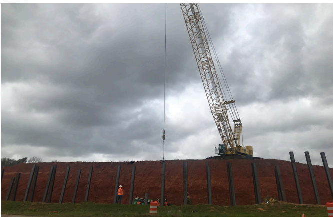
Crews driving piles for the bridge over McCrary Rd.
